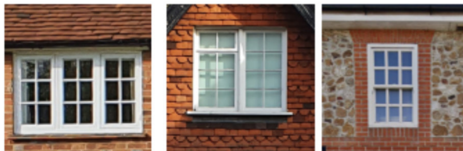
Equal mix of Cottage casement windows - with sash windows on higher profile buildings other feature windows including bow, bay and arched, on older properties the former often relate to shop fronts and display windows
