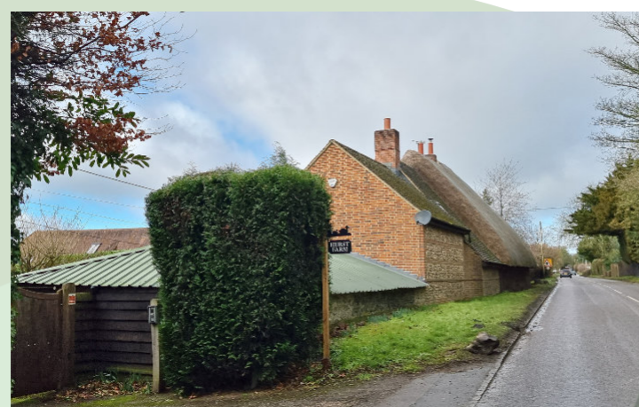
Ermin Street has many private driveways leading directly on it. This means that vehicles stop suddenly, particularly delivery vehicles and often obstruct the road
