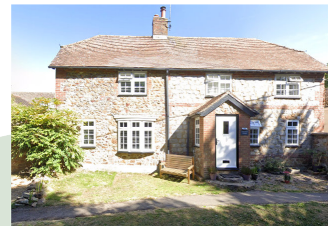
Interest can be added to the street scene by the use of contrasting materials, through projected elements and combining dwellings types and outbuildings. The preference is to combine buildings rather than make a single dwelling unnecessarily complex.
