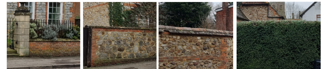
Low brick wall topped with railings
