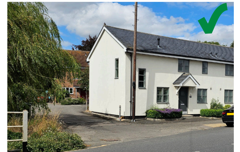
Here, a pair of old cottages has been refurbished with high quality materials and contemporary window placements to the side. The proportions of the original windows and doors have been retained. Small personalisation strip front gardens have been provided
