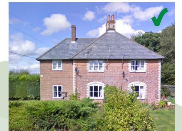
The extension of this cottage follows the original form of the dwelling with a subservient addition. The ridge line is lower, as are the eaves and it is set back from the main body of the dwelling. It successfully complements the dwelling without competing. Whilst it could be argued that the brickwork detailing should match, it could also be argued that the same level of detailing would compete with and detract from the original property
