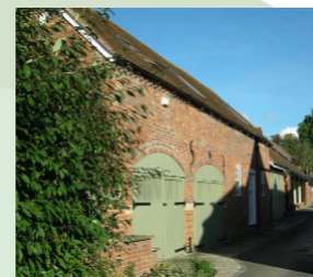
Successful retention of existing openings allow the original use to be read
