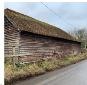
Traditional timber cladding and clay tile roof
