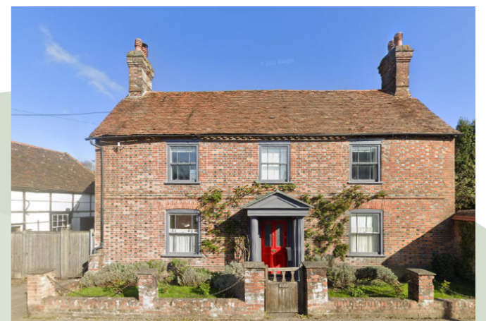
Decorative ridge detailing is commonplace. Ridge tiles are often a same colour to the roof tiles.
