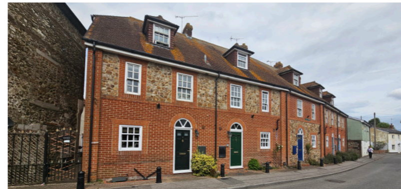
Lion Mews (adjacent to the former Red Lion Hotel) on Newbury Street is a good example of redevelopment utilising high quality materials and design detailing which reflect the local character of the area.
