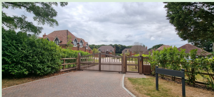
Here an example of how a new executive, gated development to replace previous single bungalow set in large grounds.
