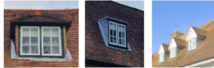
Small cottage casement dormer windows, generally set into the roof with some cutting of the eaves line. Simple form detailing or decorative bargeboards. Dormer windows are small, non
