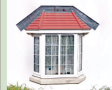
Preformed bay window canopies in GRP with poorly coloured roofing and excessive use of flashing is not in keeping with the character of the area
