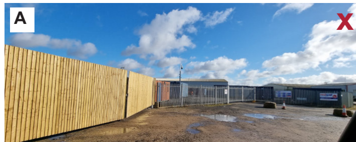
Image A shows unpainted palisade fencing and close board fencing which are inappropriate in the North Wessex Downs.
