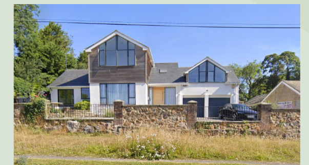
Extended to a now 1.5-2 storey dwelling of an original design with interesting detailing and materials
