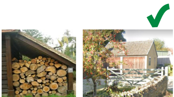
A simple overhang or catslide roof on the edge of an outbuilding can form an effective log store
