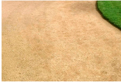
Compacted self-binding gravel
