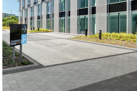
Concrete flag paving to building entrances
