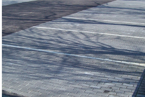
Concrete block paving to car park bays
