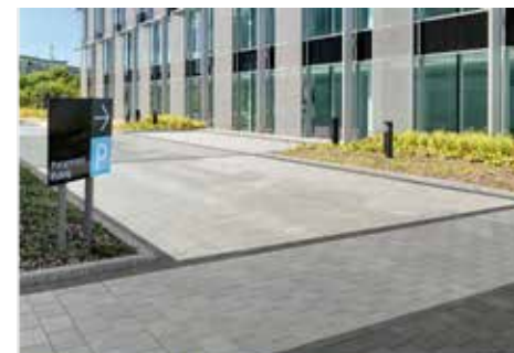
Concrete flag paving to building entrances
