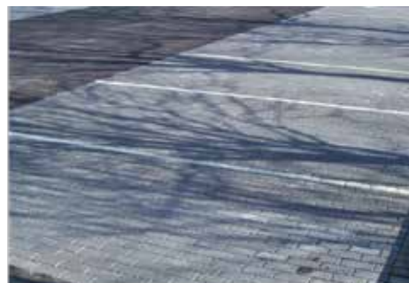
Concrete block paving to car park bays
