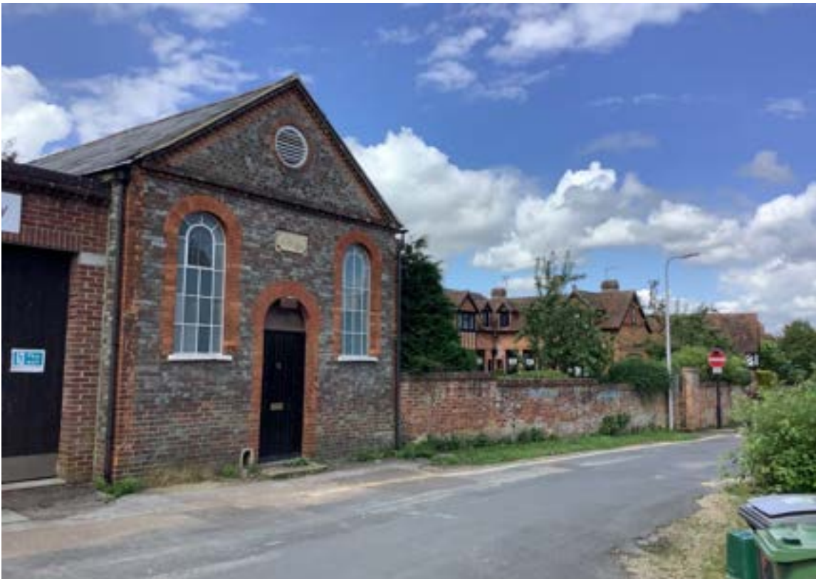
Figure 239: Unlisted building, former Wesleyan Methodist Chapel in burned brick on Hampton Road.
