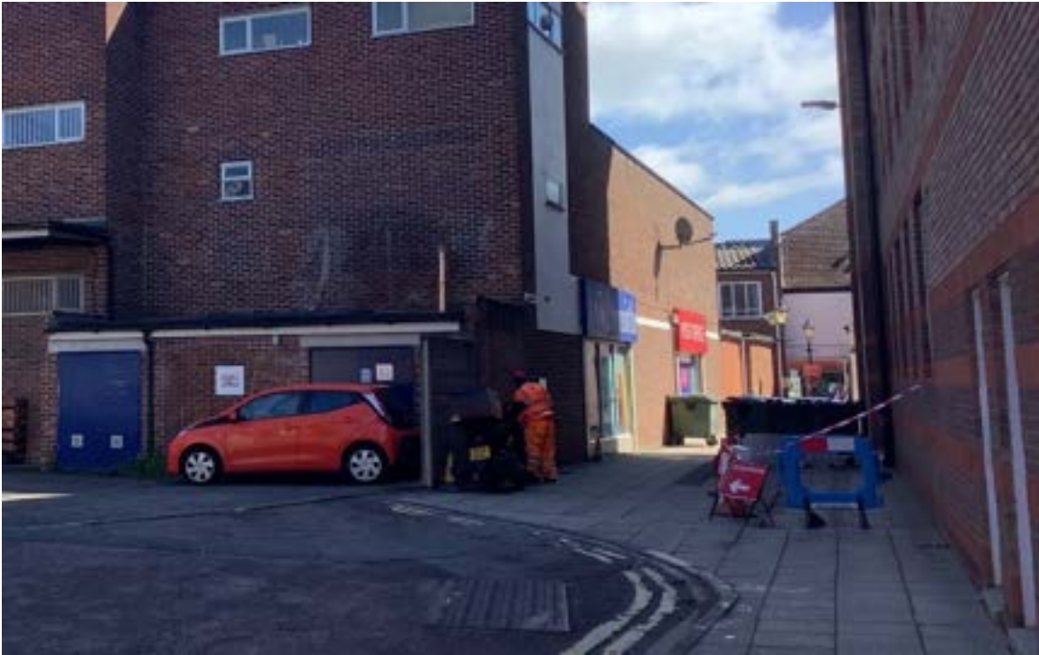
Figure 37: Passageway connecting Pembroke Road with Northbrook Street, which has been co-opted for bin storage.
