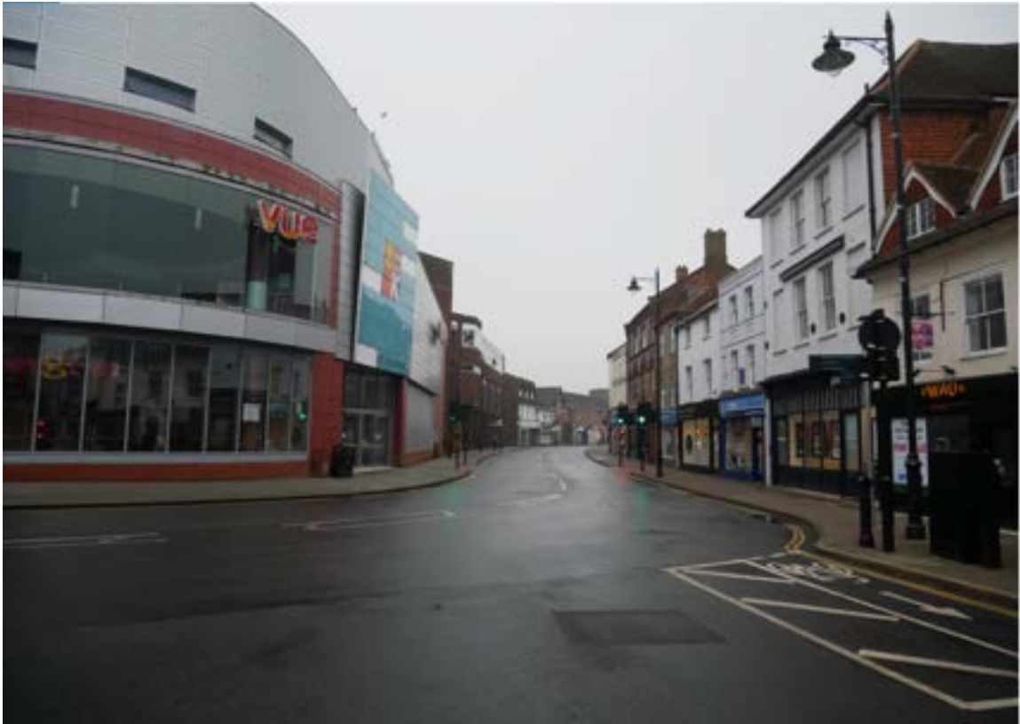
Figure 114: The Vue Cinema, part of the Kennet Centre. The form, features and materiality have made no reference to the historic context.
