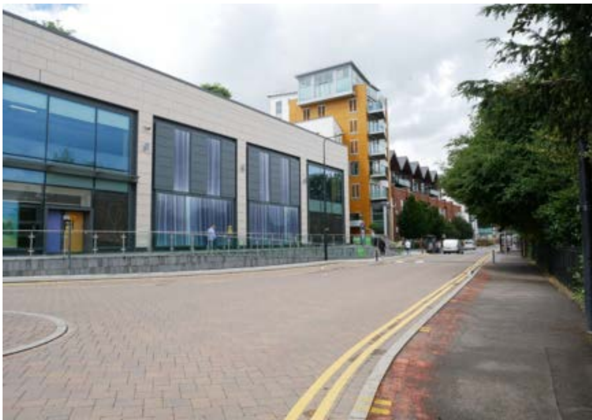
Figure 136: Parkway development showing the former John Lewis 'Home' department store and the modern setts on the southern part of Park Way.
