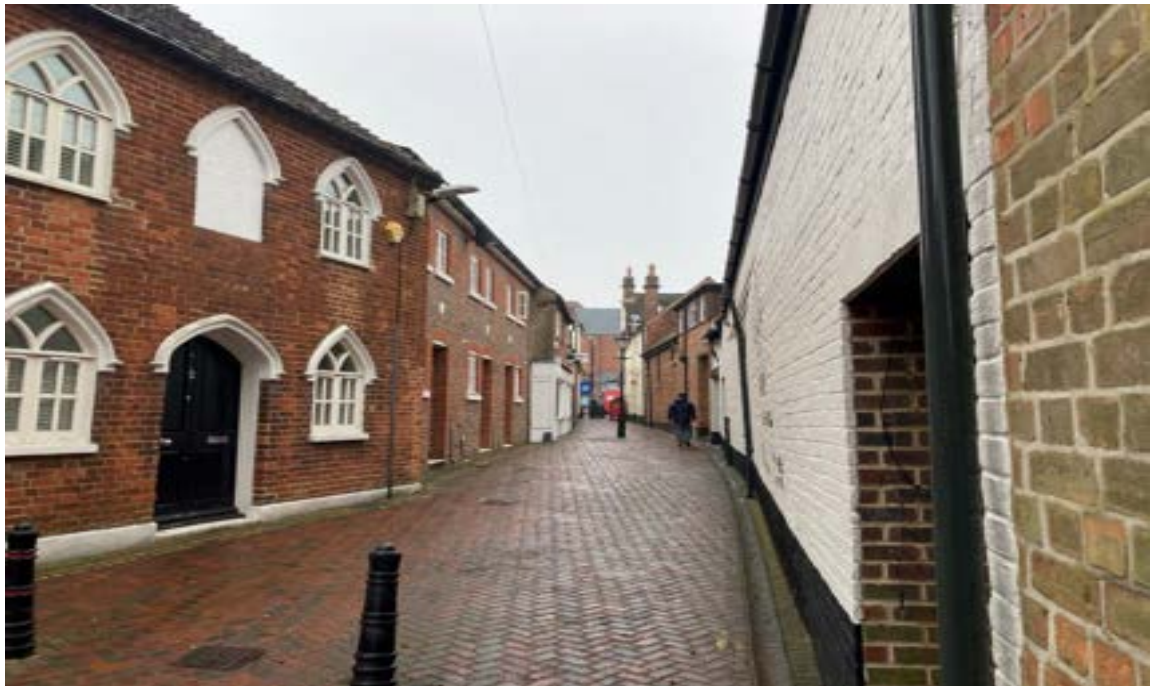
Figure 104: Inside the Conservation Area. Looking east towards Northbrook Street west, provides a sense of the deep plot pattern, undulating route network, historic fabric is visible.
