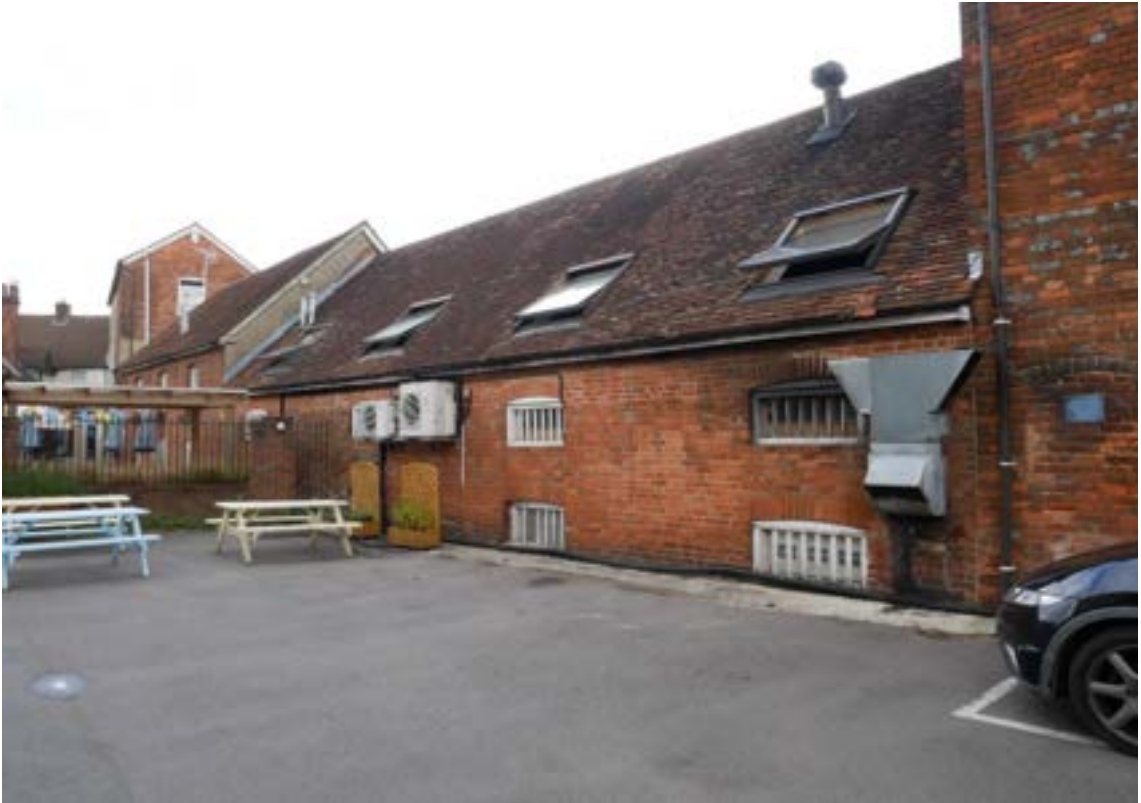
Figure 44: Void space behind the buildings on Inch's Yard. The space has been partially used for pub seating by the Dolphin Pub on Bartholomew Street, and partially used for parking.
