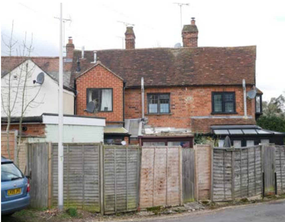
Figure 121: Poor quality boundary treatment on Derby Road. The building has unattractive satellite dishes and boiler flues.
