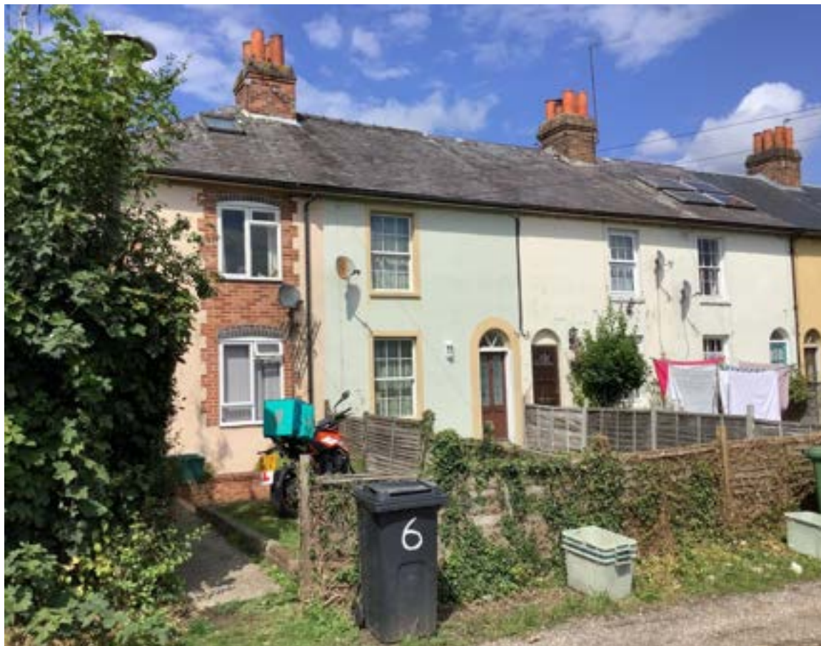
Figure 242: Grade II listed terraced houses on Madeira Place.
