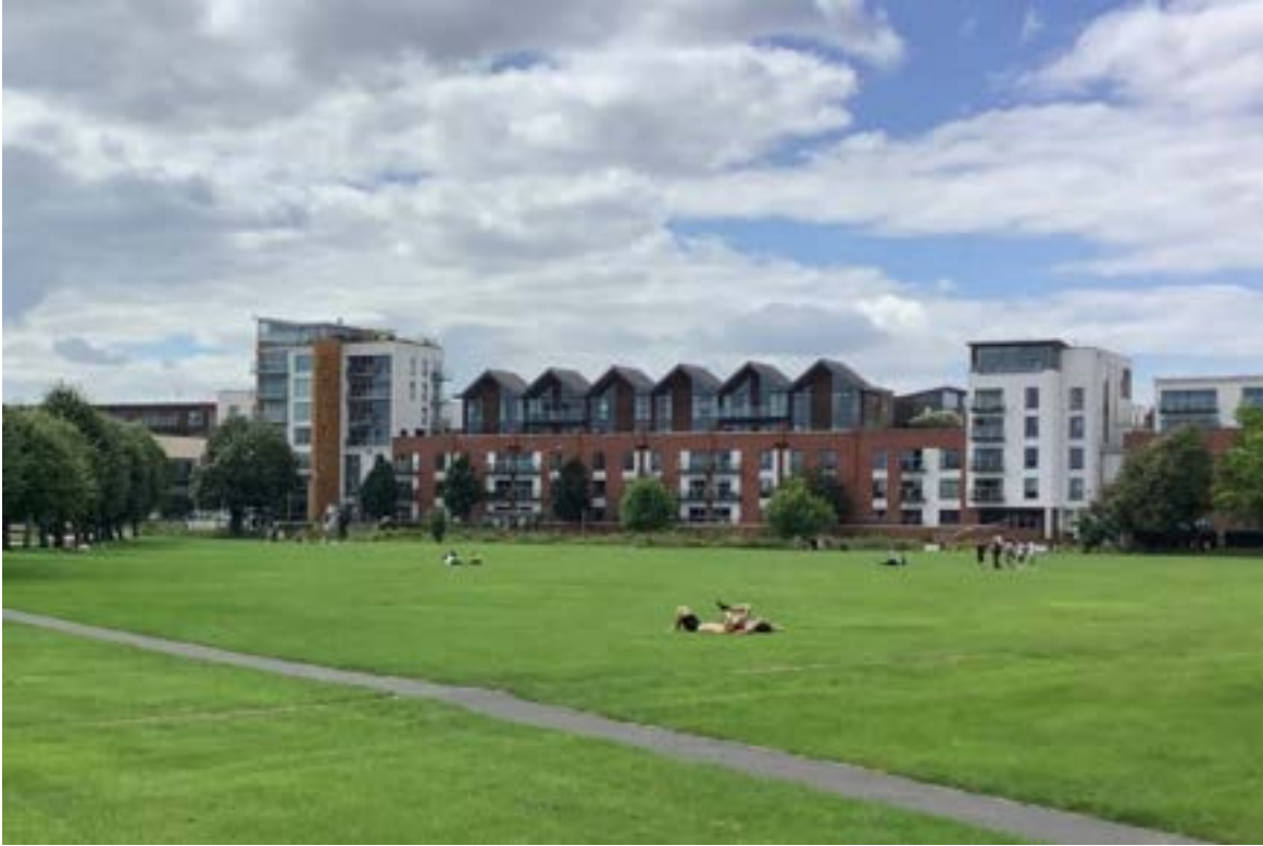
Figure 139: View towards the modern residential development on Park Way including the tallest element on the northwest corner of Marsh Lane.
