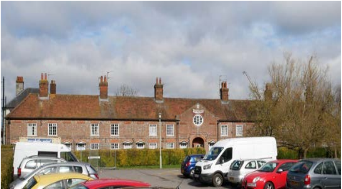
Figure 235: Lower Raymond's Almshouses on the east of Newtown Road.
