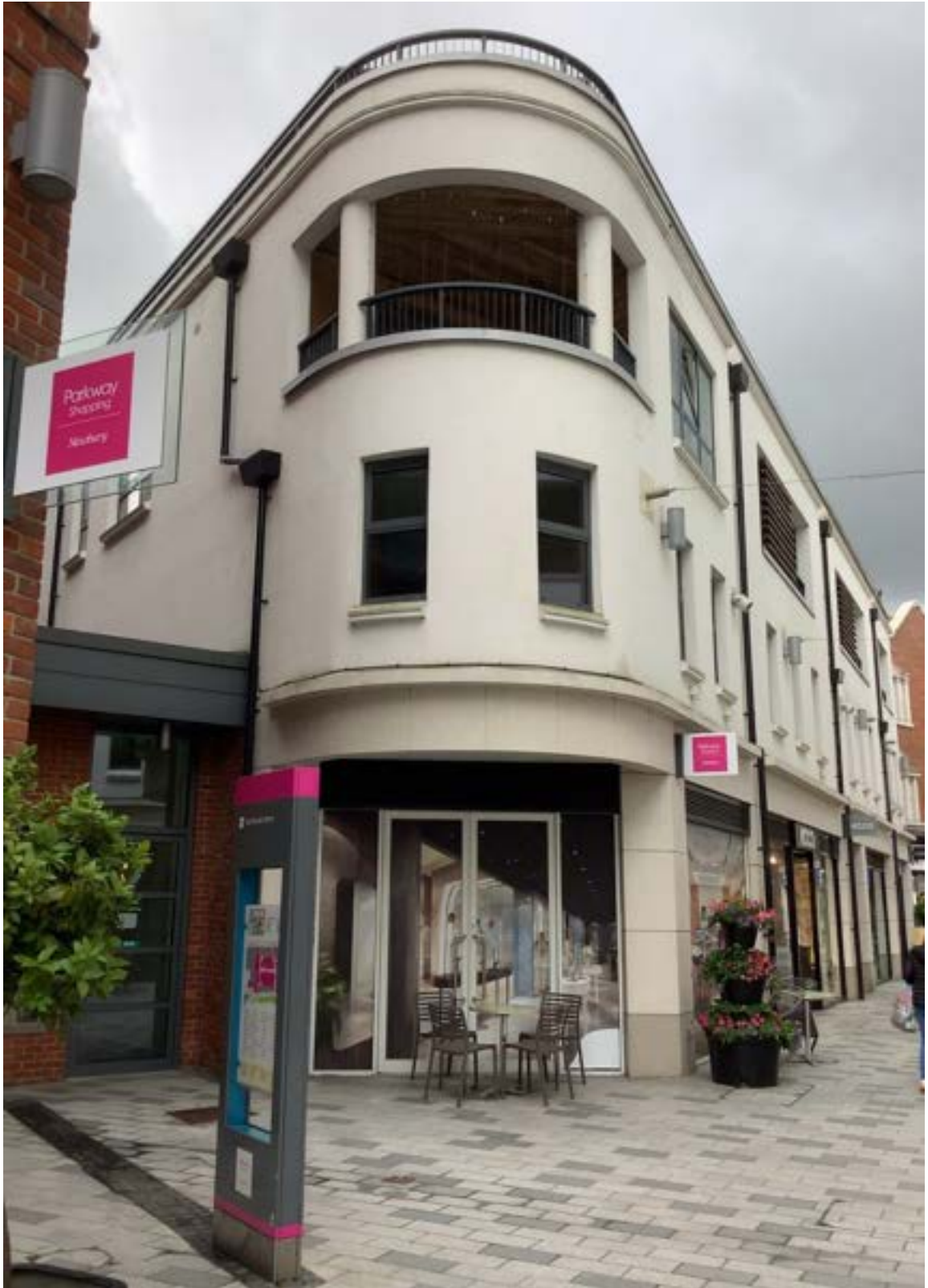
Figure 140: Corner building on West Street within the Parkway shopping area.
