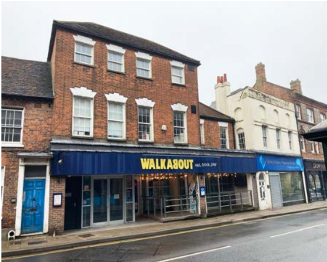
Figure 120: Shopfronts, such as this one on Cheap Street, are overly dominant and detract from the historic character of the buildings.
