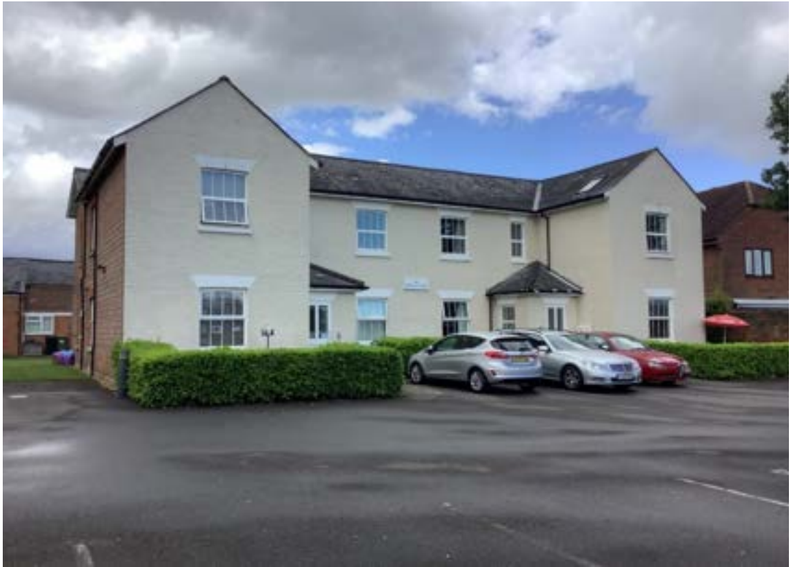
Figure 187: Car parking area in front of the 19 th century Old Police Station, now converted into flats.
