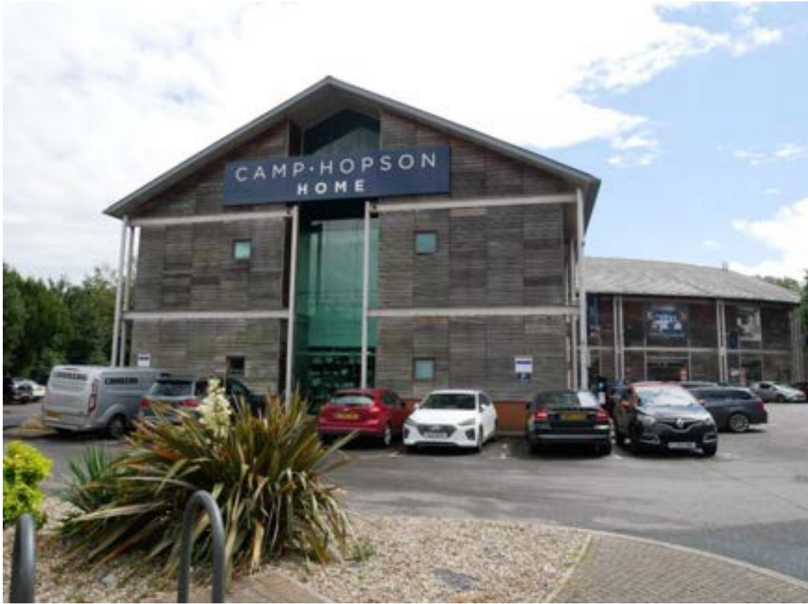
Figure 141: Camp Hopson 'Home' building in the southern part of the character area, which backs onto the canal towpath to the south.
