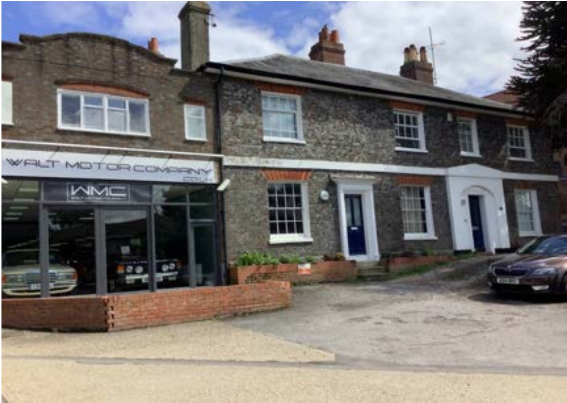
Figure 240: Grade II listed villas in burned brick (right, 22 and 24 Newtown Road) and adjoining early 19 th century addition (left, unlisted).
