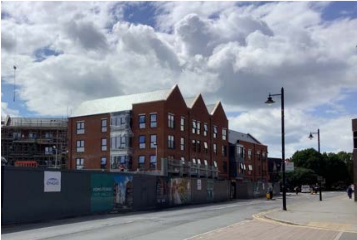
Figure 201: Weavers Yard residential development (under construction).
