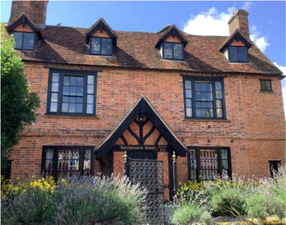
Figure 237: 4 Argyle Road 'Bartholomew Manor' Grade II listed, originally a hall and solar, dendrodated to 1436.
