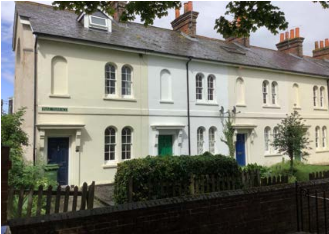
Figure 130: Listed Buildings of Park Terrace which overlook Victoria Park on its northern edge.
