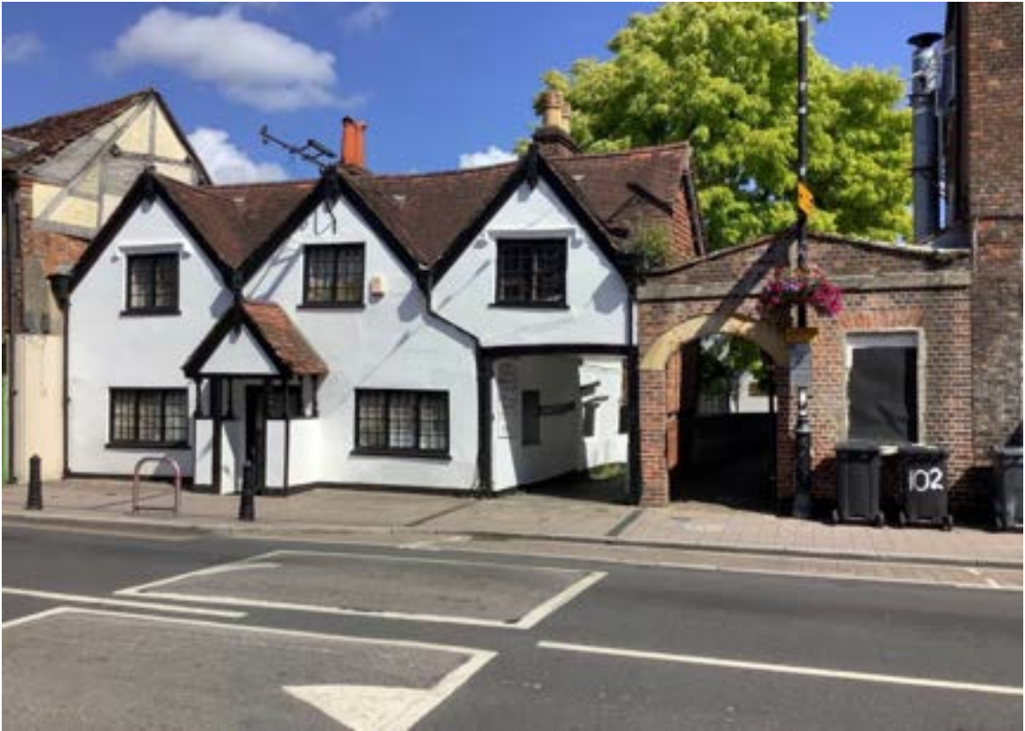
Figure 214: The Eight Bells, former public house (Grade II listed) with front facing gables and an over carriageway above Eight Bells passageway.
