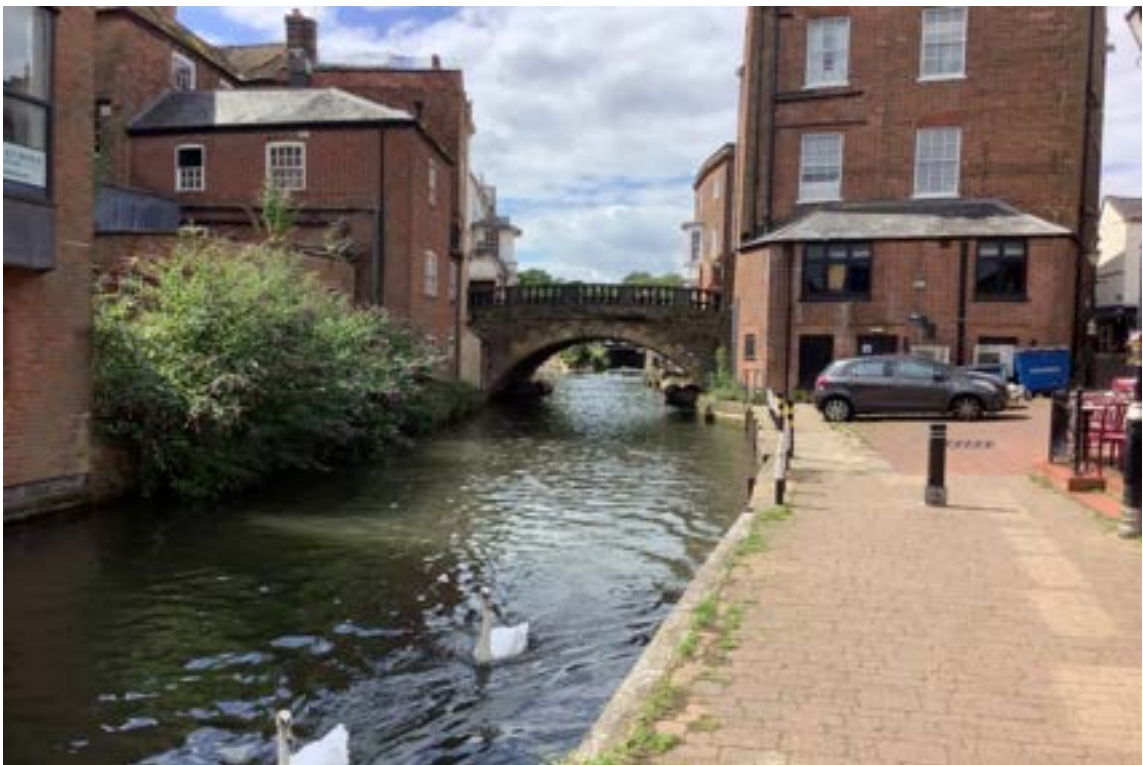
Figure 76: Representative kinetic viewpoint from outside of Newbury Town Centre Conservation Area looking into the Conservation Area towards Newbury Bridge, which is a focal point of this view and a local landmark. The rear of historic buildings in the town centre provides a sense of dense urban development. Newbury Bridge forms a key focal point and landmark.
