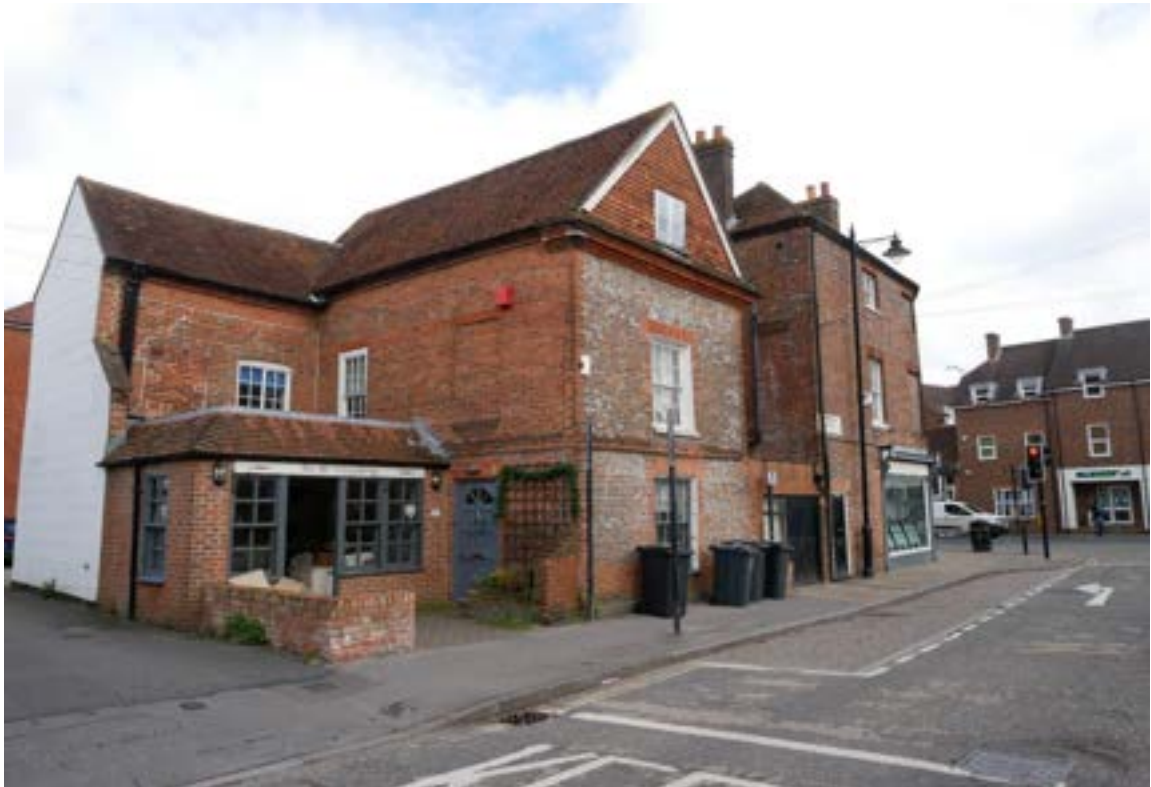
Figure 223: Grade II listed The Garden House on north side of Pound Street, a residential building with an historic shop attached.
