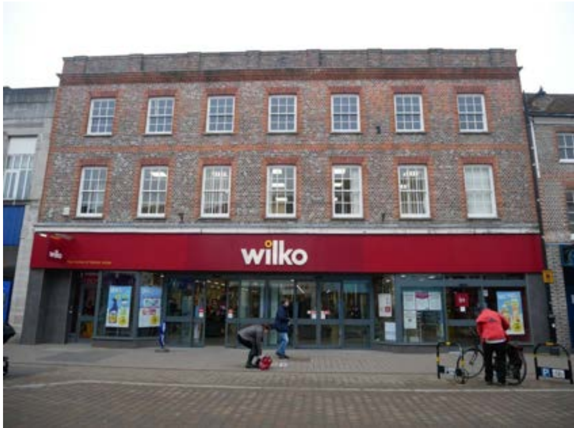
Figure 155: 13 – 15 Northbrook Street, built 1959-60. The red branding of the fascia and modern shopfront at ground level is overly prominent even on this large building, which is seven bays wide.
