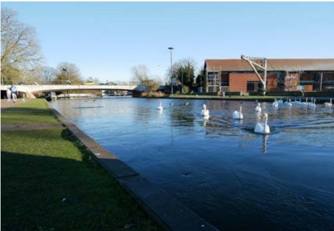
Figure 48: Southern extent of Victoria Park – view across the canal eastwards and towards the Wharf area.
