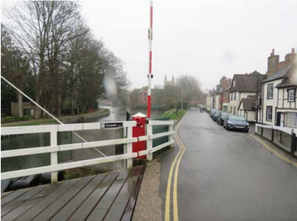
Figure 82: Representative kinetic viewpoint outside the Conservation Area looking east along West Mills from the bridge with St Nicholas' Church Tower a visible landmark, experienced in the context of the canal and its associated land and infrastructure.
