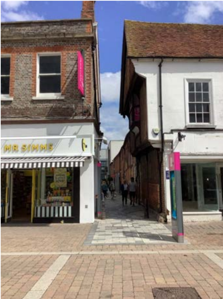
Figure 106: Inside the Conservation Area. Marsh Lane from Northbrook Street looking east, provides a sense of the deep plot pattern. Historic fabric is visible, giving public access to the historic fabric along the side of 24 Northbrook St (“Jack of Newbury’s House”)
