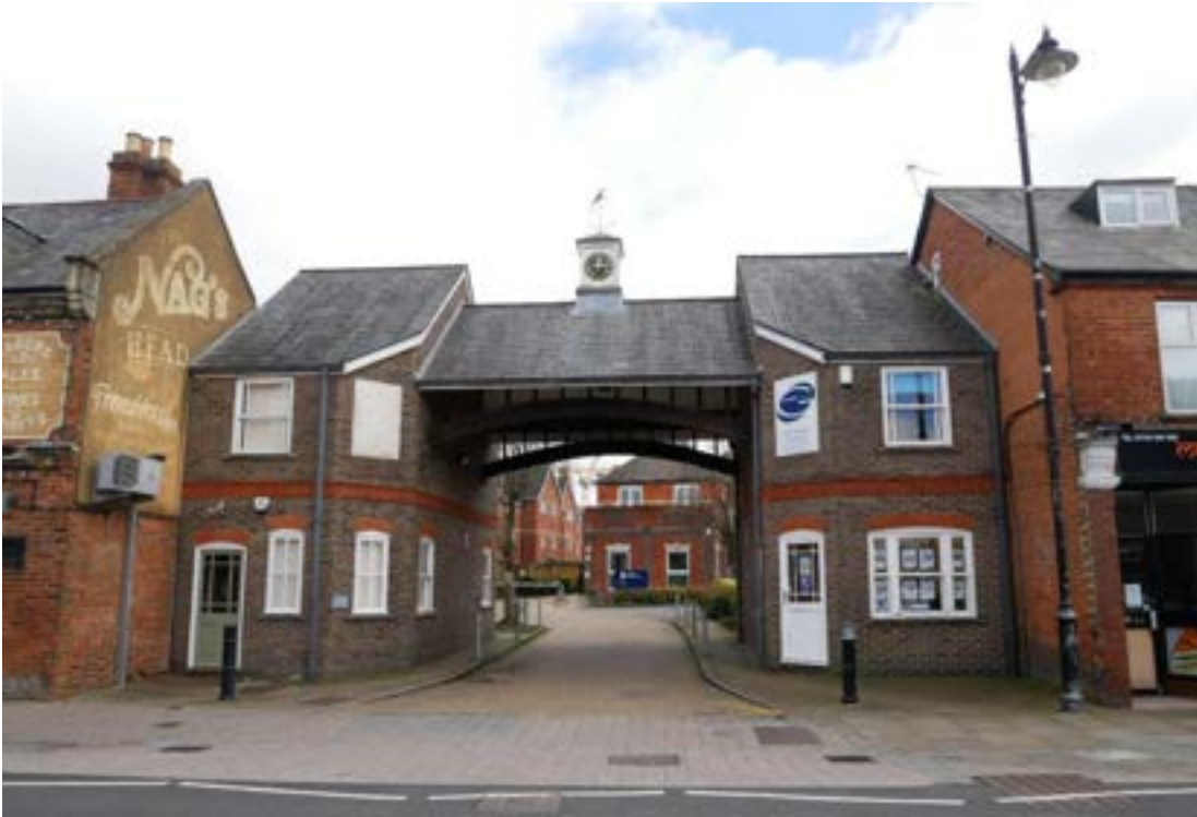
Figure 17: A modern building referencing the carriageway motif at 90 Bartholomew Street, offering a visual break in the streetscape through to the courtyard beyond.
