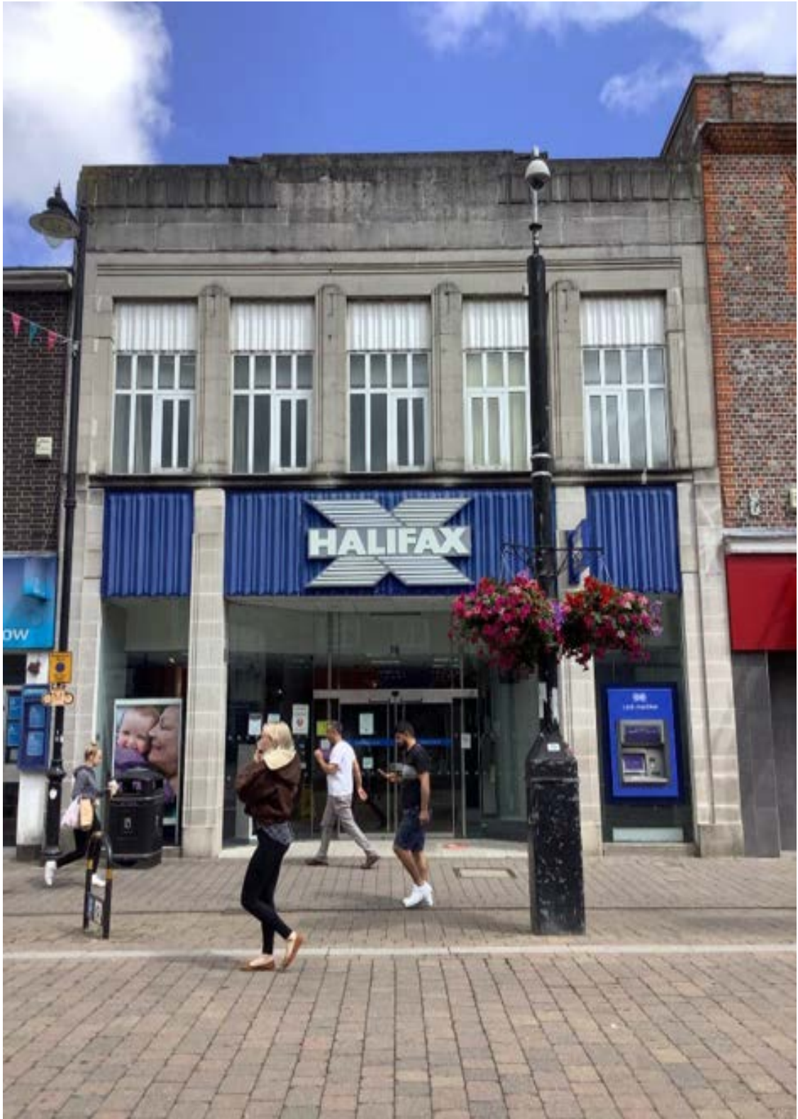
Figure 164: 16 Northbrook Street, an early 20 th century Art Deco building, somewhat anomalous in style but reflecting the varying ages of the frontages in this character area.
