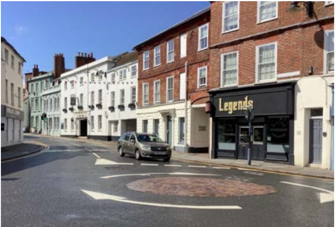
Figure 171: View looking west along Oxford Street from the Broadway junction. Numerous buildings have large carriageway openings indicating their former use as coaching inns.
