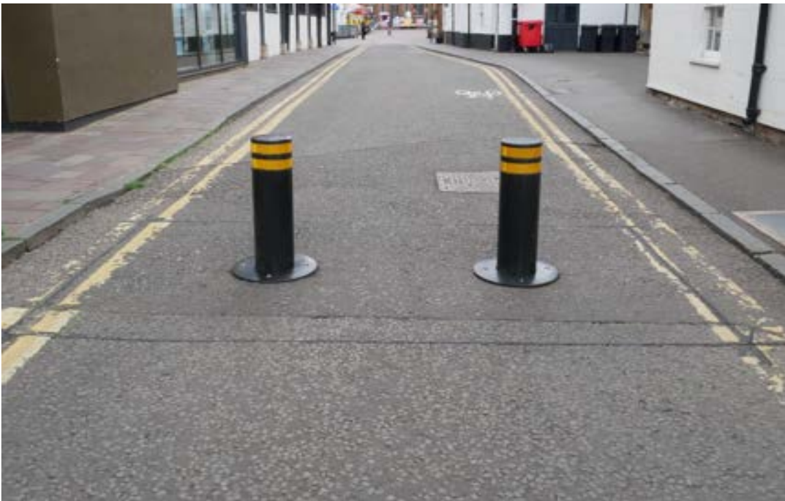
Figure 26: Raising bollards on Wharf Street (in the Kennet and Avon Canal (East) Conservation Area), preventing vehicular access into Market Place during traffic restricted hours.
