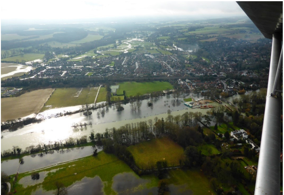
Pangbourne during the 2013/14 flooding
