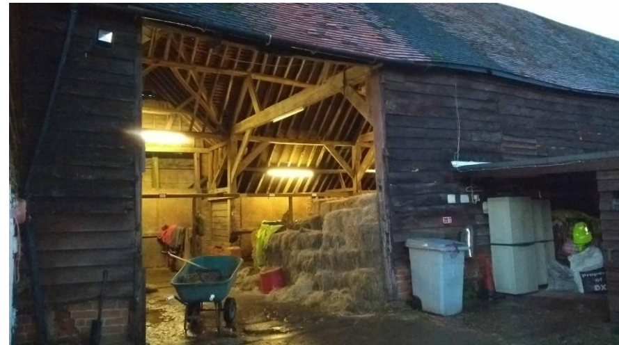
Figure 8 interior of the great barn showing timber construction
