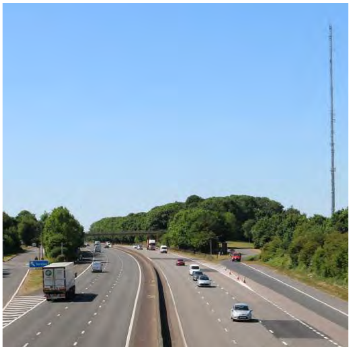
M4 motorway, Membury Services and telecomms mast
