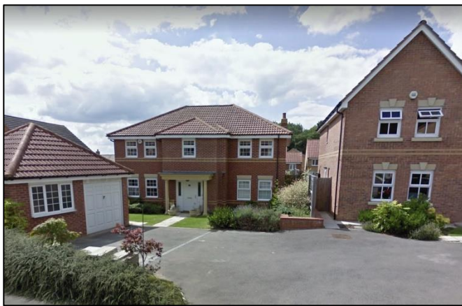
Modern housing in the north-east part of Newbury – the style is in stark contrast to the Villages Zone
