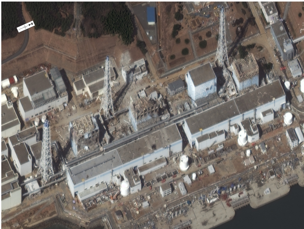
Figure 8: Post Accident Photograph of Reactor Units 1-4 at Fukushima-1
