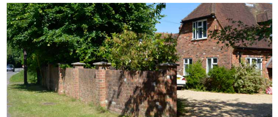
Brick wall with piers along residential property frontage on Reading Road
