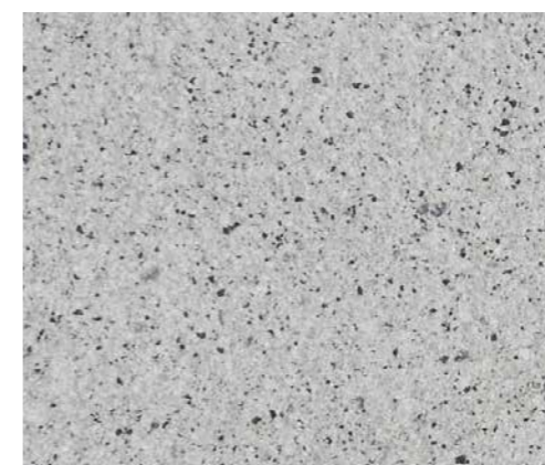
Textured Concrete kerb with granite aggregate
