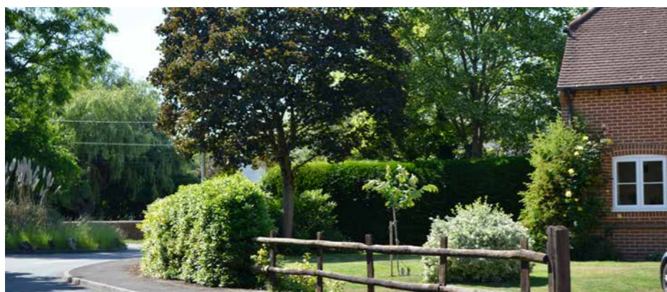
Property boundary treatment using timber post and circular log rail fencing on Hillside
