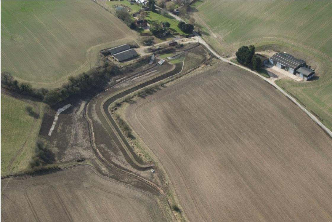
Figure 4-7: Winterbourne Flood Alleviation Scheme (photo credit: West Berkshire Council)
