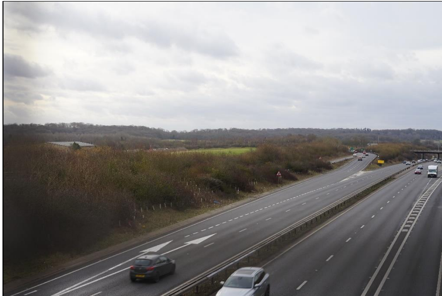
Photo 3: Long view from Priors Court Road to site, just visible as open field below wooded horizon
