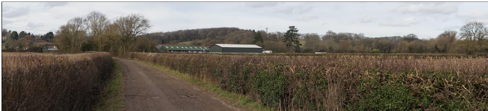
Photo 3: View from Clay Lane (PRoW: BEEN/1/7) over managed hedgerow to the right (site boundary), with an agricultural barn visible against the buildings within one of the fragmented PEAs, with the Kennet Valley side beyond (January 2022)
