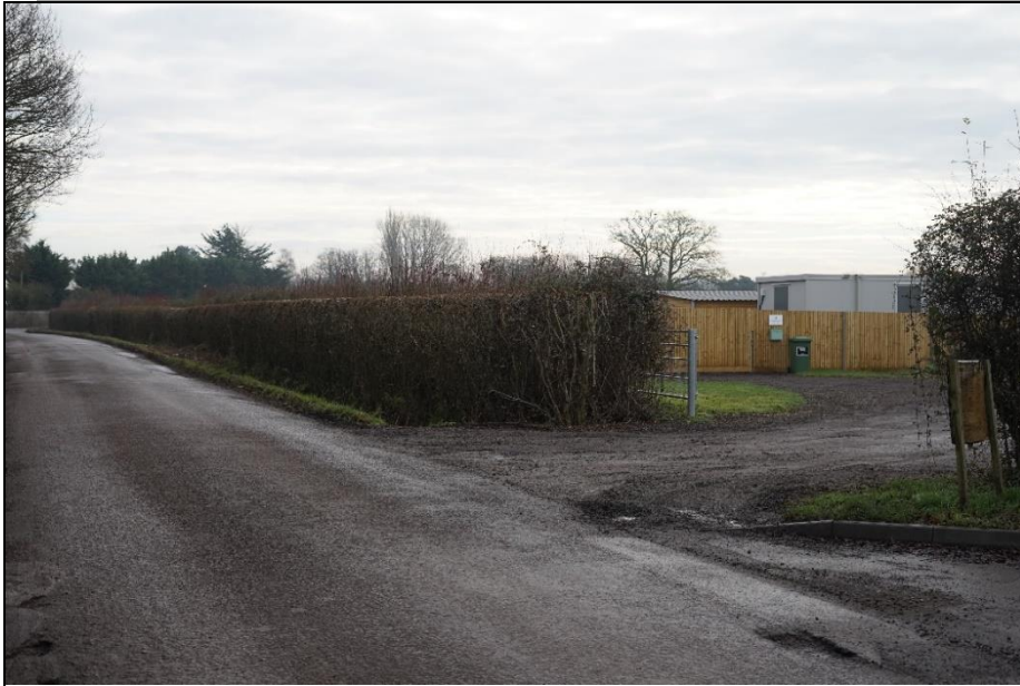
Photo 9: View of field entrance to site from Grange Lane (PRoW: BEEN/17/4), showing the temporary portacabins for The Woof retreat – dog day-care
