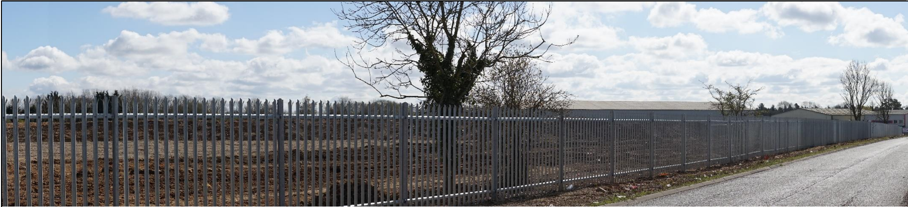
Photo 8: View into site, with site boundary marked by grey palisade steel fencing, occasional tree with earth bund beyond. The highway tree planting on the skyline is just visible. The building within the adjacent PEA is also visible, located at a slightly lower height
