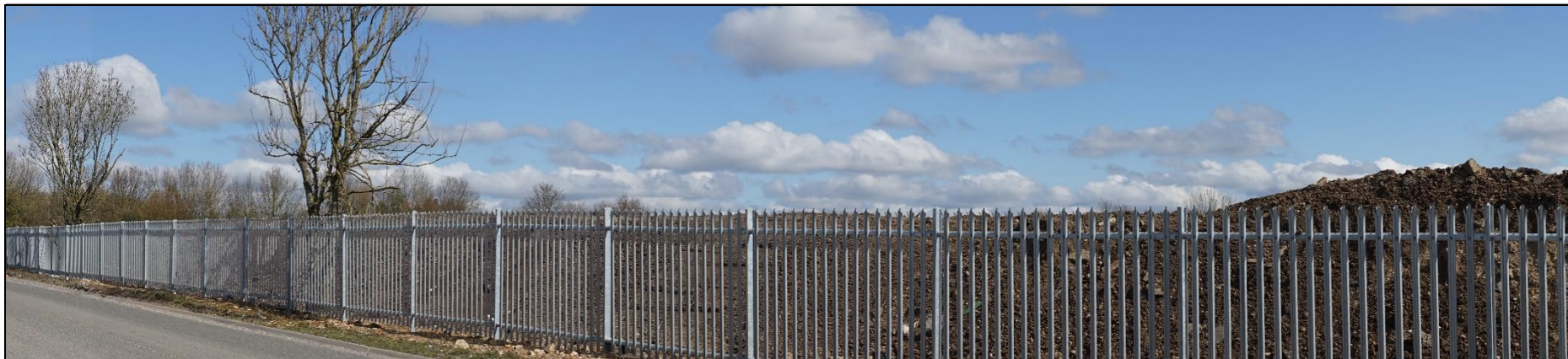
Photo 6: View into site, with site boundary marked by grey palisade steel fencing, occasional tree with earth bund beyond. The highway tree planting on the skyline (which aligns the northern and north-eastern site boundary) is just visible
