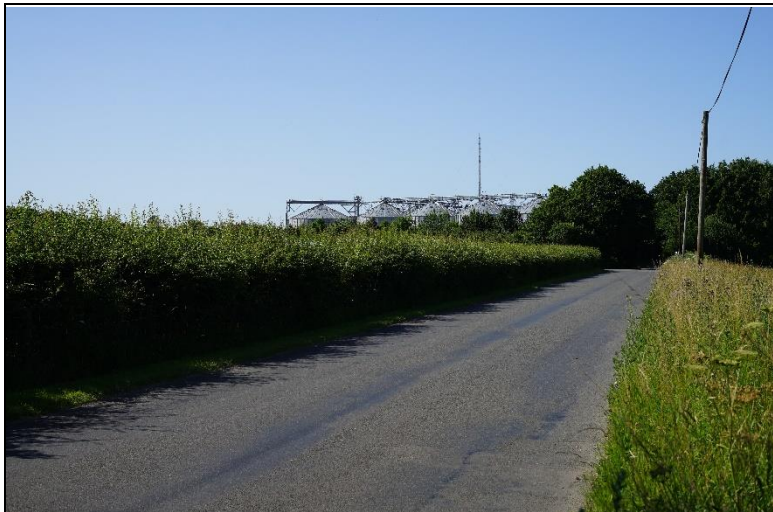
Photo 3: Looking north with site beyond field hedgerow to left. The tops of the silo towers are visible (within PEA) above intervening maturing woodland (July 2021)
