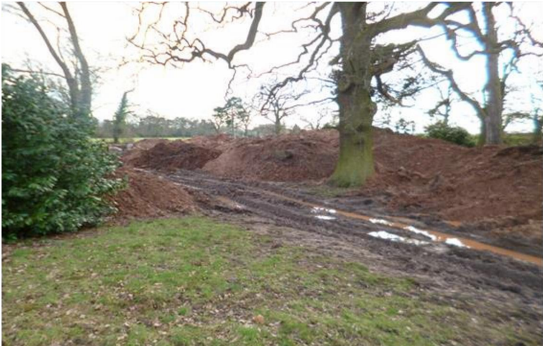
Damaged soil structure from the passing site vehicles within the Root Protection Zone.
