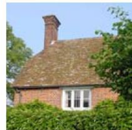
Stoke. Traditional casement window and chimney detail.
