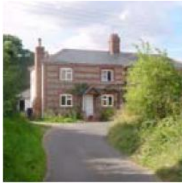
Egbury. Bands of brick and flint are a feature of many vernacular buildings.
