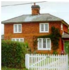
Stratfield Saye. Distinctive casement windows.
