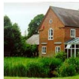
Bradley. Traditional materials and interesting detailing on a relatively new property overlooking the village pond.
