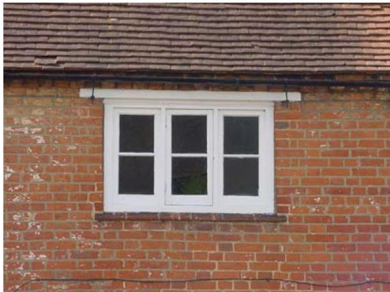
A typical casement window in a vernacular red brick and clay tile house, Old Basing
