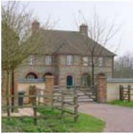
Brown Candover. An individual style of flint and brick house with a hipped roof.
