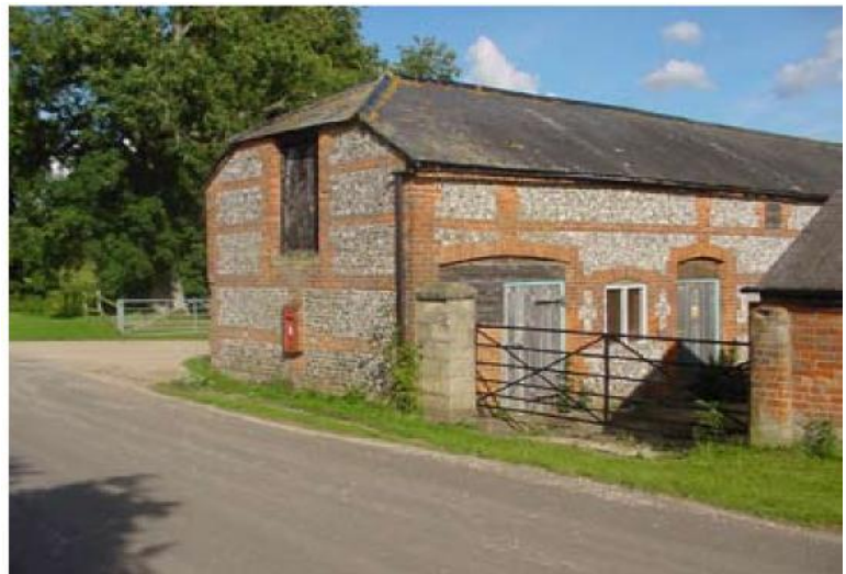
Brick and flint farm building with a half-hipped slate roof, Egbury
