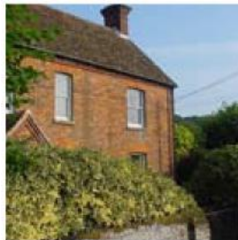
Stoke. Traditional sash windows and a low brick boundary wall.
