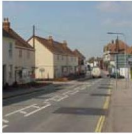
Overton. Infill terraced houses in the village centre give continuity to the street scene by picking up on local building styles and scale.
