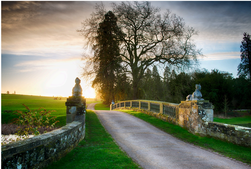
Photograph 6: Carriageway and ornamental bridge at Kington Lacey
