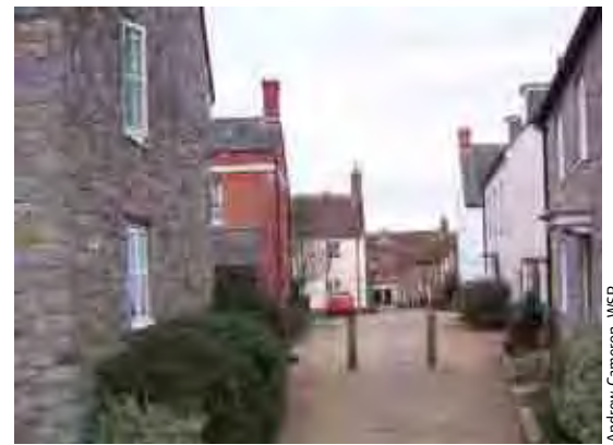
Figure 4.9 A good example of a pedestrian/cycle route at Poundbury, Dorchester. It is short, direct and with good surveillance.
