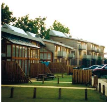
Solar panelling on house roofs in Berkshire
