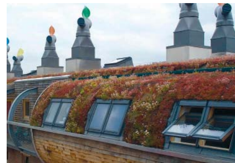
Green Roof on house at BedZed
