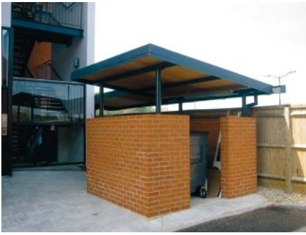
Well designed bin storage located at the back of the block
