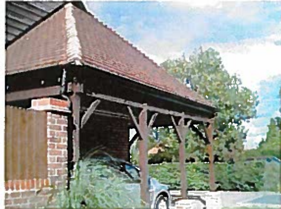
Covered parking space at Ingles Edge
