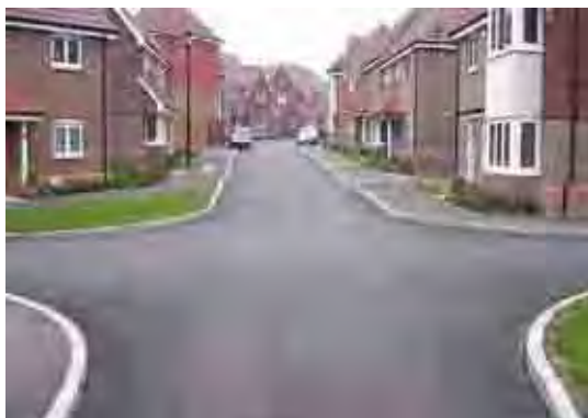
Figure 9.5 Four-way junction with no marked priority.
