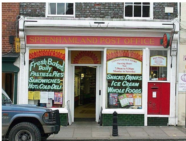
This Victorian shopfront is full of interest and includes details such as the original blind, glazed tiles and interesting corbel details
