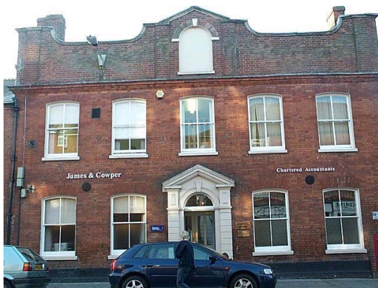
A fascia sign on this building would be inappropriate. These applied letters convey the message whilst retaining the character of the building
