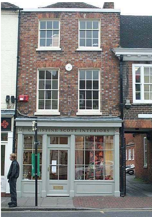
This modern shopfront follows the basic classical principles and respects the proportions of the overall building
