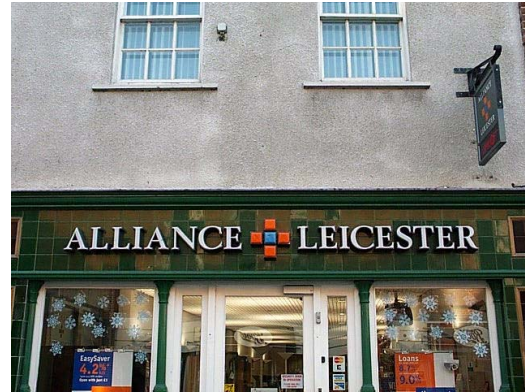
This lettering has replicated the shiny ceramic background of this interesting historic shopfront to good effect
