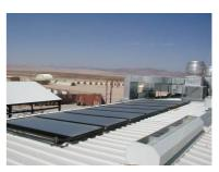
SHW systems are well suited to domestic properties and can provide up to around 65% of DHW demand. To correctly situate the panels there should be sufficient roof space for their installation with a preferably open SE-SW facing roof and sufficient space for hot water cylinders close to the panels.
