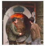
Biomass boilers are designed to allow modulation of the output down to about 30% of optimum output, however, for efficient and economic combustion biomass should be burned frequently at high temperature and as such it is common practice for biomass to be supported by conventional gas boilers to meet peak demand periods<sup>9</sup>.
