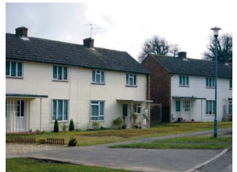
Post war local authority housing, Burghfield Common
