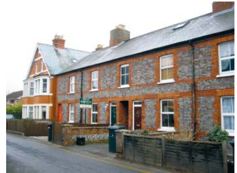
Red brick used to highlight key elements of the frontage composition
