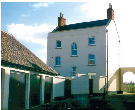
Parking courtyards can be accommodated in the back of blocks and increase privacy distances
