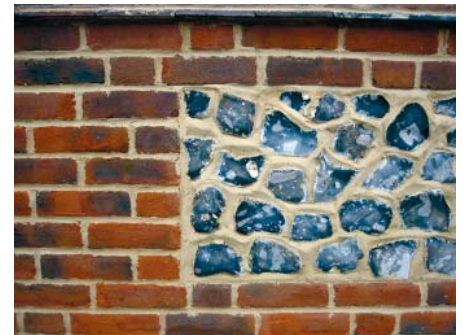
Flint is used to render elevations and walls
