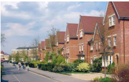
Small front gardens incorporating driveways within new development
