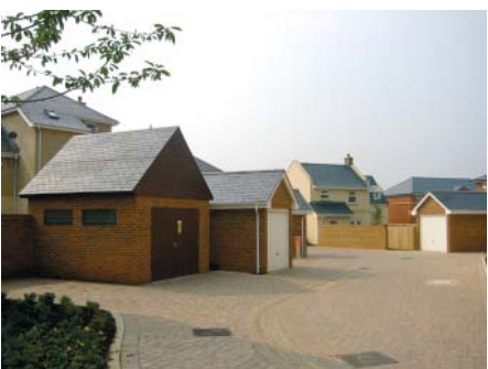
Parking courtyard located at the back of a new housing block
