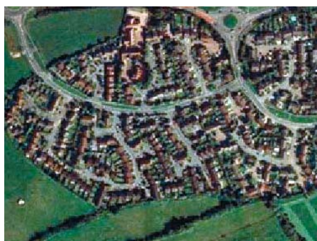
Less permeable 1980's distributor road and cul de sac layout at Calcot
