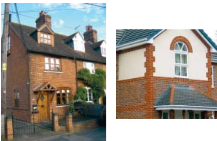
Knowing what traditional building materials are used within an area can help inform design proposals
