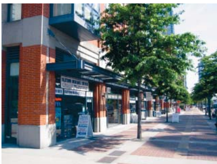
Ground floor mix of uses, with residential or office floorspace above add diversity to streets, enabling them to feel safe and secure
