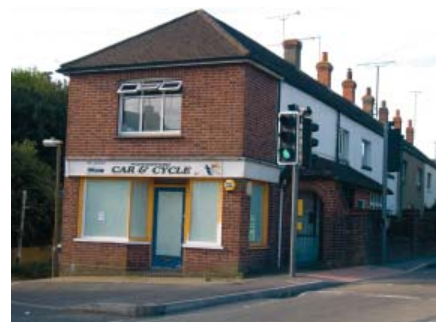
Vacant unit on Salisbury Road
