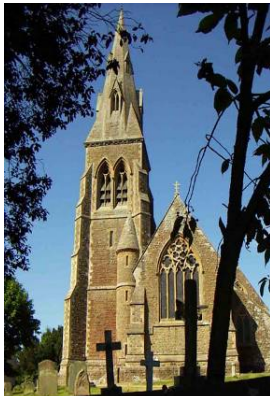
The north east corner of St. Mary’s church
