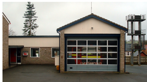
Mortimer fire station
