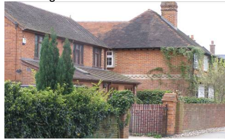
Typical semi-detached housing showing decorative coursing
