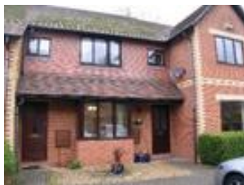
Modern housing in the Laneswood development showing decorative banding and corbelling
