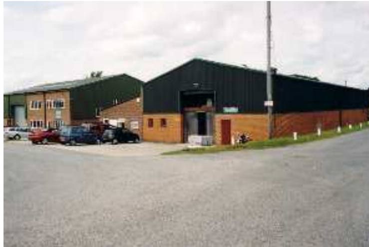
Red Shute Industrial Estate
