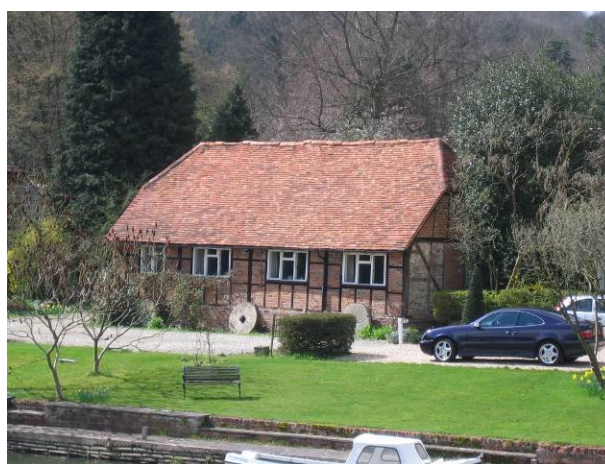
Figure 12: Store or warehouse associated with Streatley Mill
