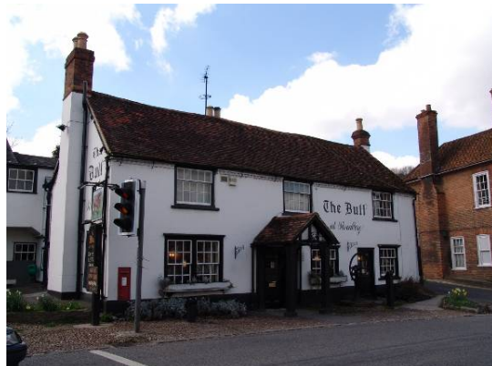
Figure 58: The Bull Inn (incorporating the Victorian post box)
