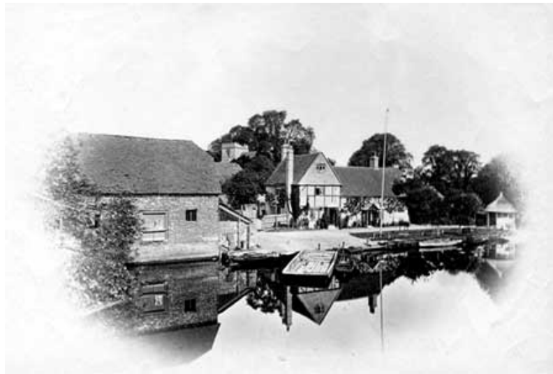
Figure 6: The Swan Inn with stables to the left in the late 1870s (HT1333, Oxfordshire County Council Photographic Archive)
