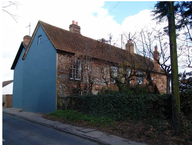
Figure 14: Townsend Farmhouse, Reading Road
