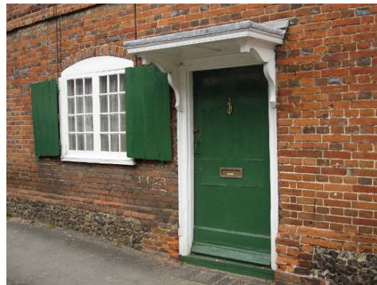
Figure 20: Casement windows, traditional shutters, door and canopy at Bag Row
