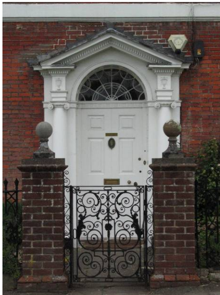
Figure 29: Entrance to Streatley House with door surround, brick piers and iron gate
