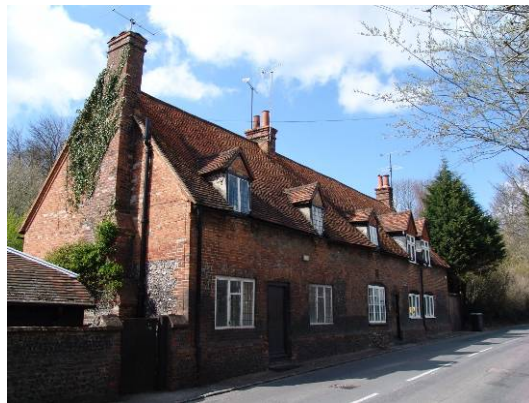
Figure 18: Gabled eaves dormers Place Manor Cottages, Wallingford Road
