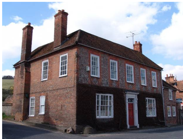
Figure 21: Panels and lozenges of grey bricks at Elm Lodge, Wallingford Road
