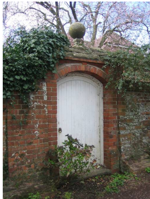
Figure 45: Door opening along Vicarage Lane
