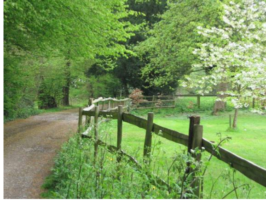
Figure 28: Timber post and rail fence at edge of village
