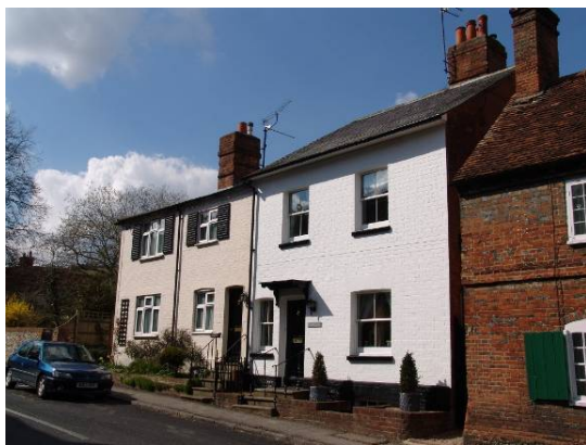
Figure 52: Coopers Cottage and Little Falklands
