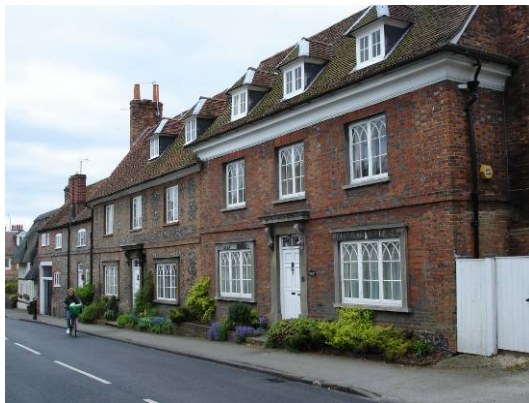
Figure 17: Dormers with hipped tile roofs Middle House, High Street
