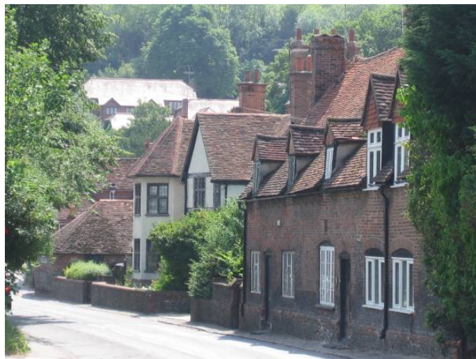
Figure 62: Roofs of the modern Hill Gardens development adversely affect the setting of the conservation area
