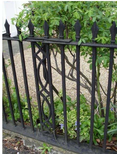
Figure 30: Iron railings at Streatley House
