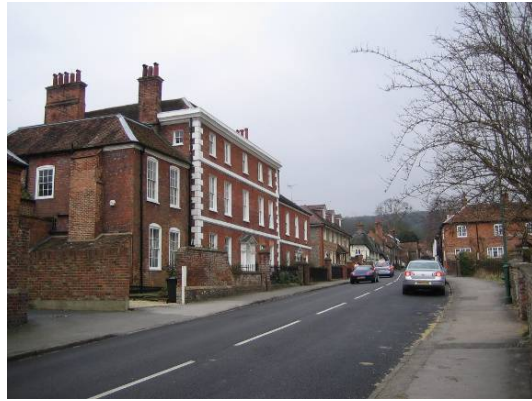
Figure 26: Streatley House provides contrast along the south side of High Street
