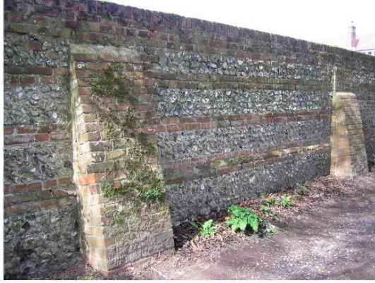
Figure 27: Flint with brick lacing courses and tapering buttresses in Vicarage Lane
